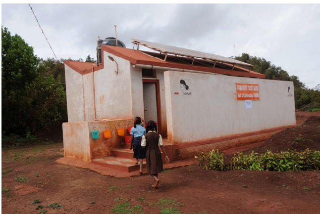
Community Toilet Block at Kammathuru Village
