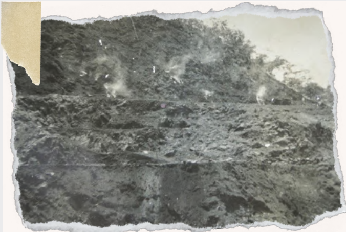
Blasting at KMK
