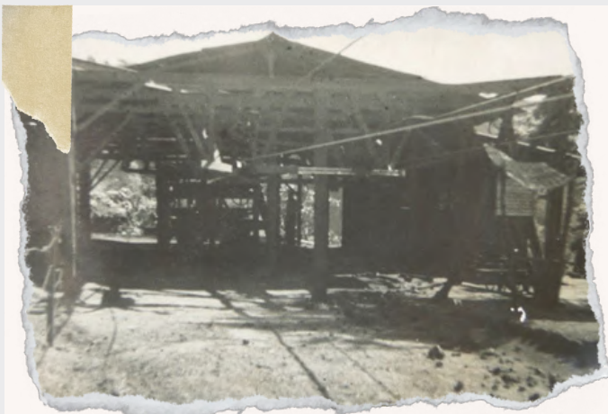
Front view of Rope way at Deogiri
