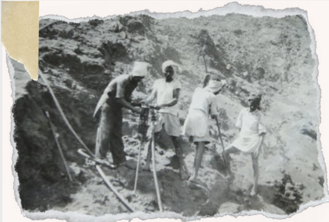
Jack Hammer Drilling at Kanige Marada Kolla (KMK)
