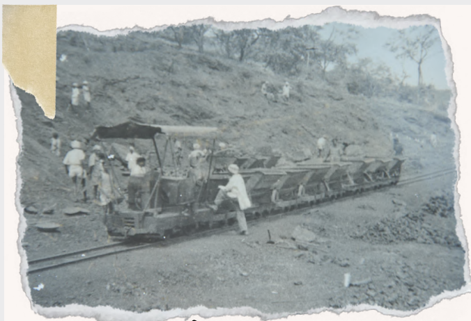
Emptying trolleys for Ore transport at Chintamana Banda (CMB)
